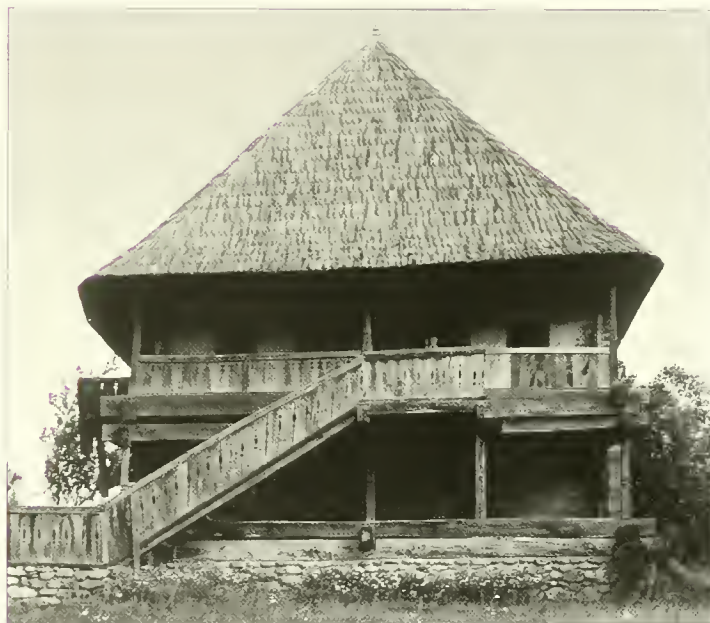
A wooden house from Gorj (18th century). Photo courtesy Village Museum, Bucharest
